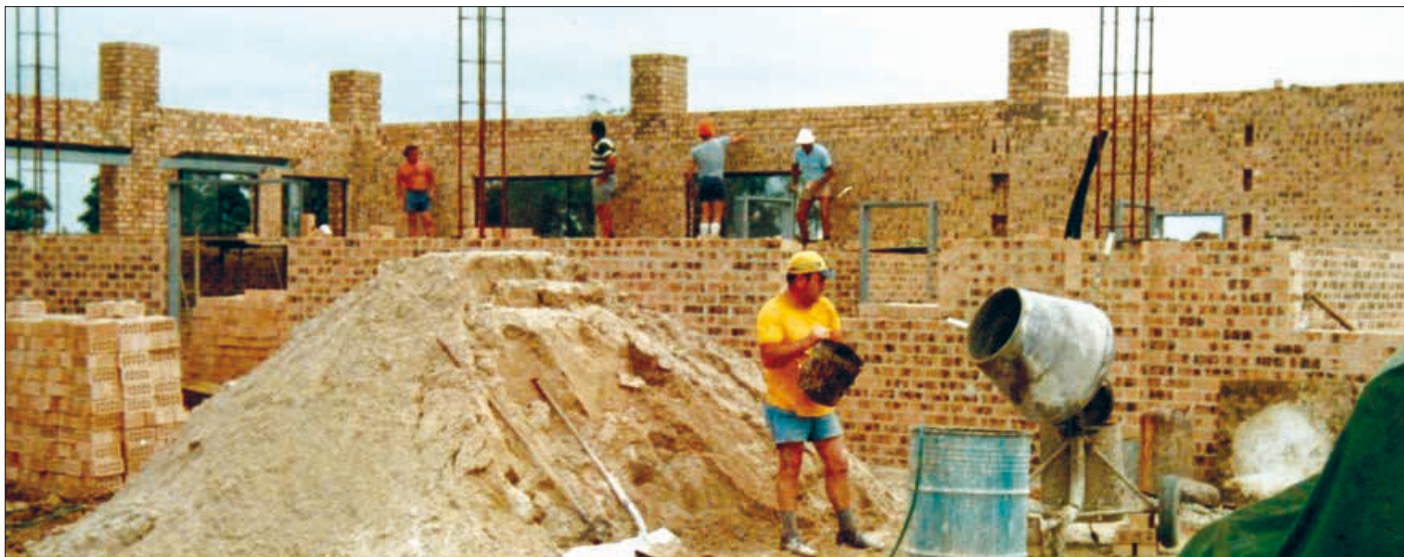
With the steel reinforcement completed, it was time for pouring the concrete
