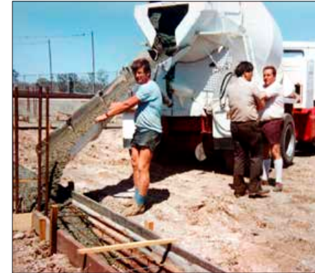
A lot of concrete was necessary. Albin Sedmak directs the flow of concrete in the foundation framework.
